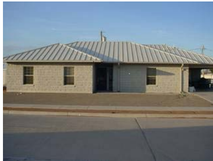
CBP Housing Unit
