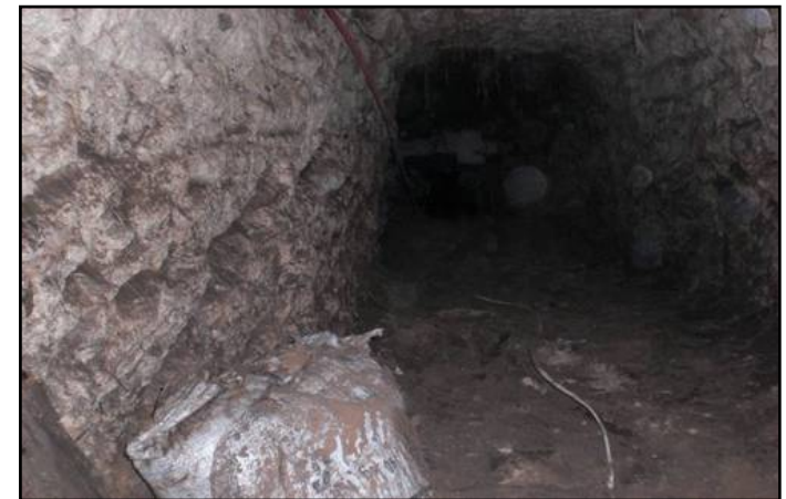
West Dunbar Tunnel
